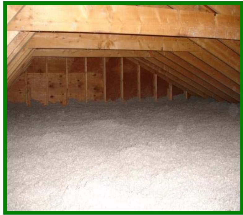
Well insulated attic after cellulose is installed
